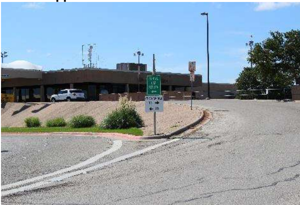
Figure 2-5 Upper & Lower Level Access Roads
