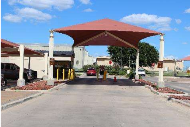
Figure 2-12 Passenger Parking Exit
