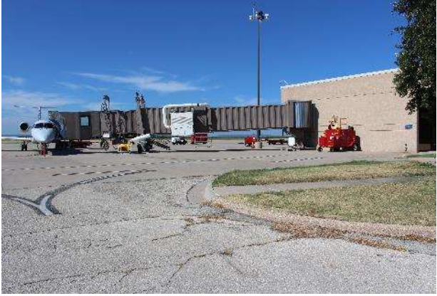
Figure 2-45 PBB at Gate 3 serving a regional jet
