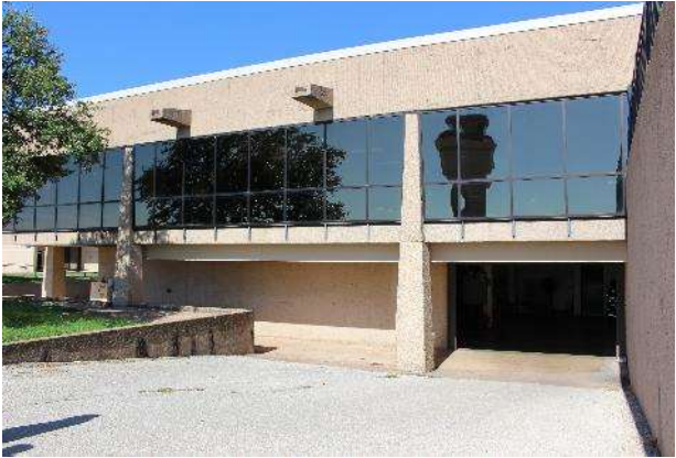
Figure 2-41 Inbound Baggage Entrance Roadway
